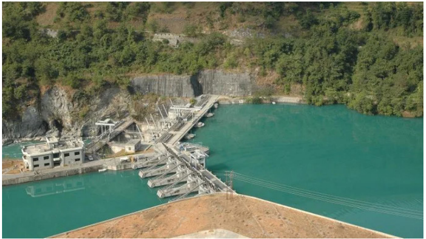
The Arun-3 Hydropower Project in eastern Nepal illustrates how large-scale hydropower development is increasingly linked to regional electricity trade and cross-border energy cooperation. Photo: Collected
